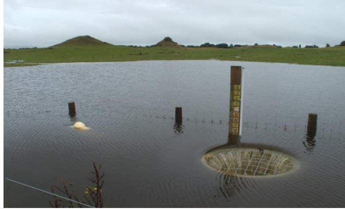
Figure 4. Upstand riser skimming uppermost layer of ponded water
