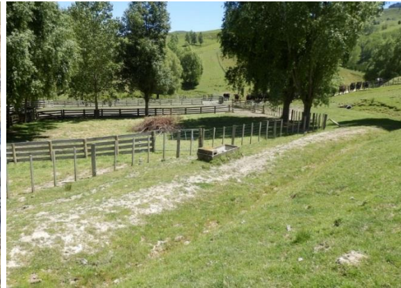
Fig.4 Diversion drain to direct upslope runoff away from yards
