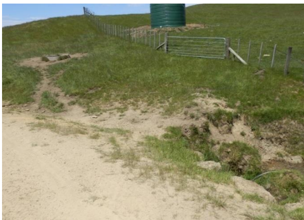
Fig. 5 Trough pad flow path to track drain, and culvert intake at bottom right of photo; landowner elected to move trough to low risk site nearby.
