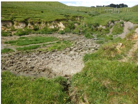
Fig. 9 Farm dam with high level of sediment deposition: actions include managing sediment at source, removal of sediment and potential modification of dam with baffles and filtered outlet.
