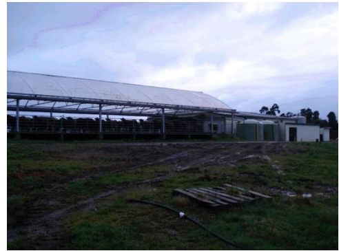
Figure 6. Covered yard, near Lake Brunner, West Coast with complete rainfall diversion. Cows are housed prior to entering the parlour
